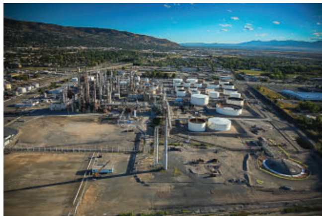
HollyFrontier Corp. has entered an agreement in principle to sell newly built crude, FCC, and polymerization units at its 45,000-b/sd Woods Cross refinery in West Bountiful, Utah. Photo from HollyFrontier.
