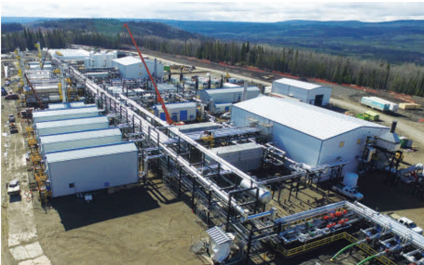
AltaGas Ltd. has fully commissioned the first phase of its Townsend integrated mid-stream complex in northeast British Columbia. Photo from AltaGas.
